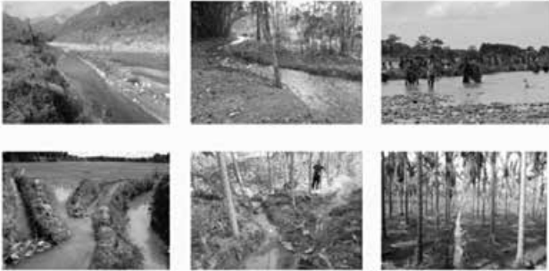
Figure 2: Diversion based dong-bandh irrigation system
